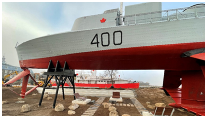
L'Escale de l'hydroptère APL (LPA hydrofoil stopover) worksite, October 2021 - Credit: Martin Bérubé, Pratte Paysage +
